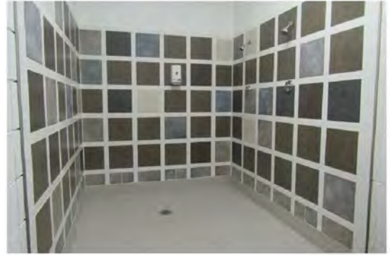
Photo #A14: Ceramic wall and floor tiles in change room shower area.
