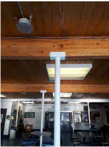
Photo #S1: Wood Beam-Steel Column in Lobby.
