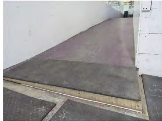
Photo #A18: Tripping hazard and lack of handrails on barrier free ramp near bleachers.
