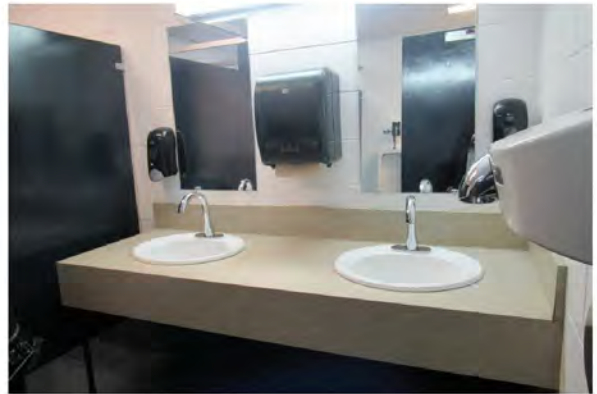
Photo #M4: Counter mounted sinks in washroom.
