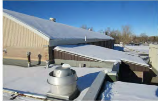
Photo #A20: Cap flashing and SBS arched roof and asphalt shingle sloped roof.
