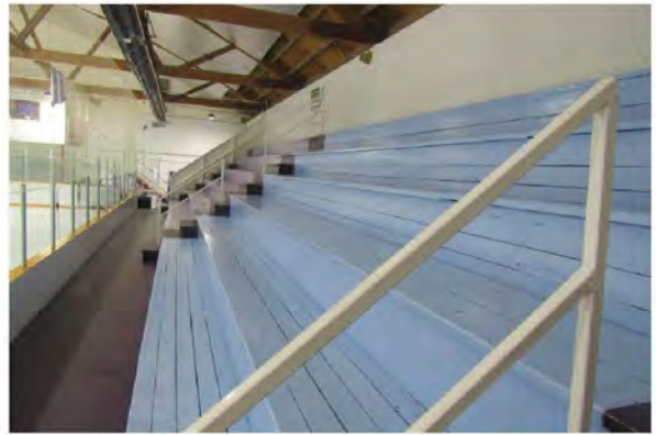
Photo #A12: Metal railings and painted bleachers in the rink.
