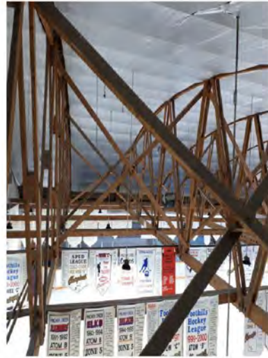
Photo #S4: Cross bracing between trusses over arena.
