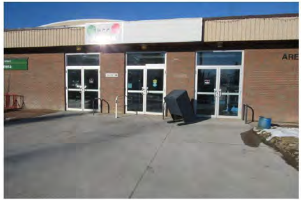
Photo #A10: Building main entrance.
