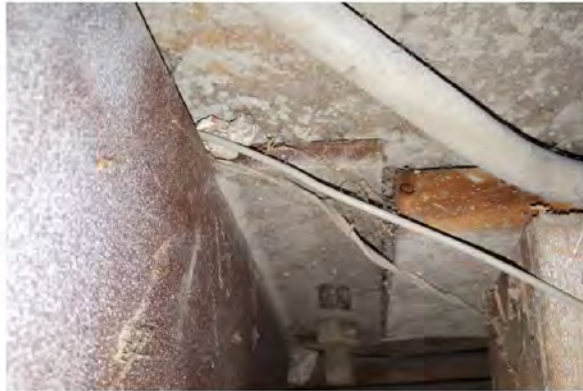
Photo #S7: Wood truss-concrete column connection.
